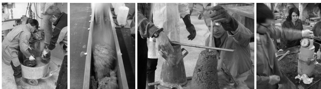
Figure 2. From left to right: concrete blending, beam casting, slump-test and air content measurement. Photos: Holger Koss.
